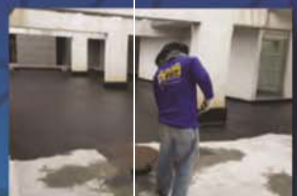
The Lake Condominium Product : Newcoat PU Roof Garden
